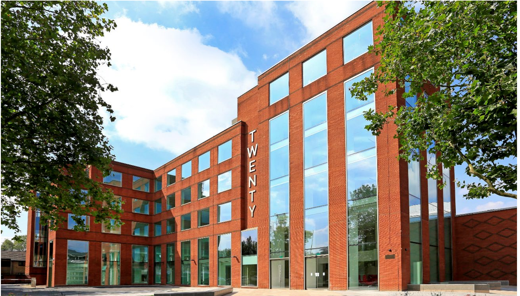
TWENTY, Staines, UK
